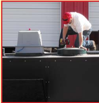
Up to 4 lift stations per unit handling 500 to 1000 gallons per day.
